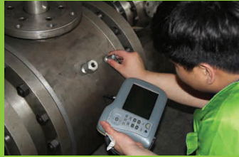
Valve Wall Thickness Test
